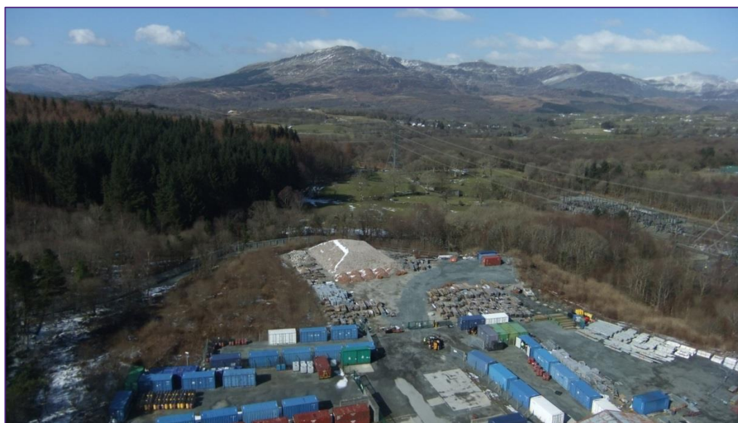
ISO Container Field and segregated waste compound
