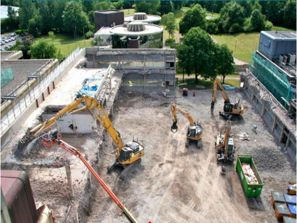
Final Site Clearance
