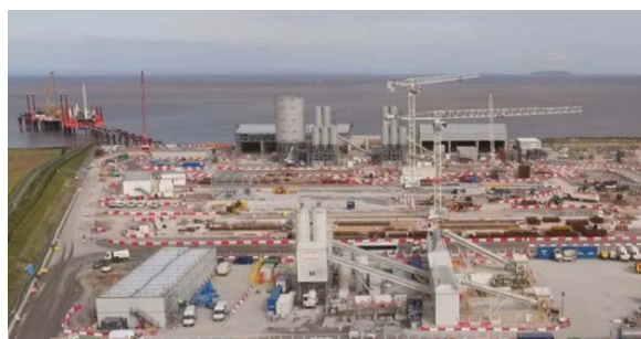
The Hinkley Point C site in September 2017
