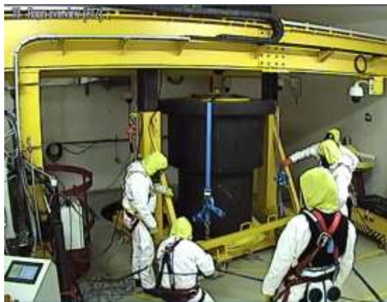
The concrete plug being lifted
