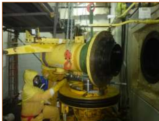
Dismantling the drive
