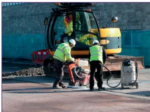
As part of the Buffer store project, a wet cutter was used as a dust suppression method. To ensure that any water slurry generated during this process did not impact surface waters, a number of measures and handling protocols were adopted. During the process a wet vac was used to collect the slurry at source, additionally booms were used to restrict the spread of any additional slurry and local drains were protected.
